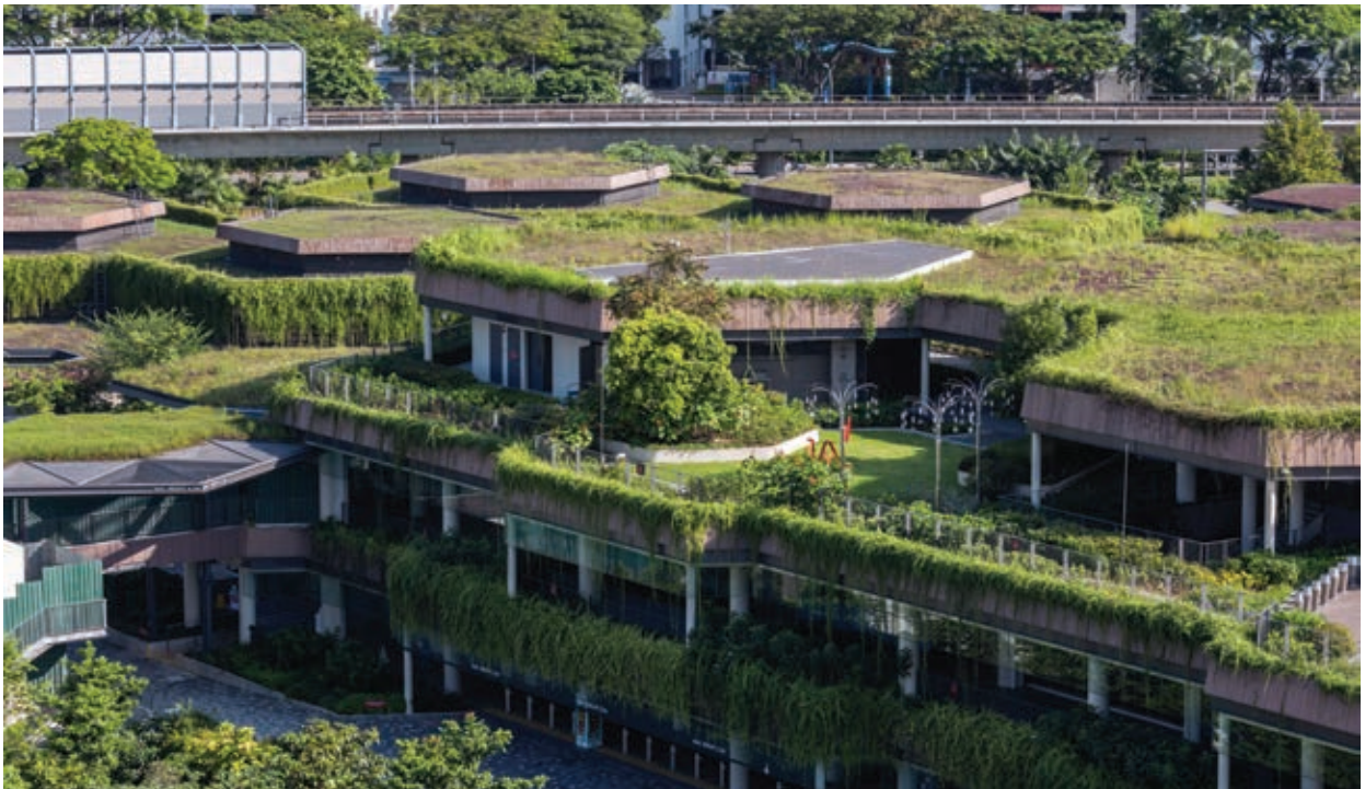
Green roof GaiaMat™ installation at the Sembawang Sports and Community Centre, Bukit Canberra. Green roof was installed by GWS Living Art in 2022 using proprietary, patented, soilless GaiaMat™ that can capture 26 litres of rainwater per square metre. Image: GWS Living Art
